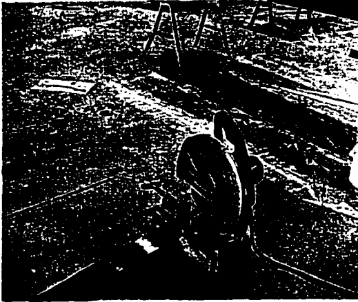
a. Cutting of CFRP plate
